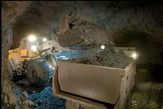
Excavation and loading place
